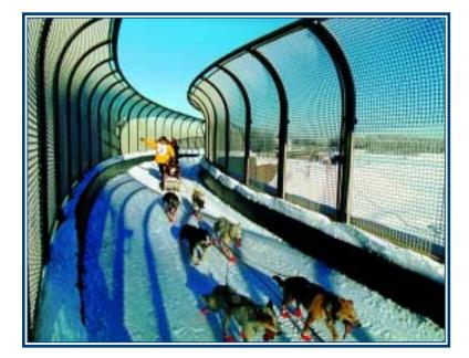
OR YEARS, THE STATE OF ALASKA AND MUNICIPALITY OF ANCHORAGE had studied ways of crossing the busy, five-lane Tudor Road with a multi-purpose trail without success. Close proximity to high voltage power lines, buried utilities, close clearance tolerances, and the desire to have a smooth, continuous crossing with grades less than 5% for use by bikers, the handicapped, and sled dog teams presented difficult design problems.
