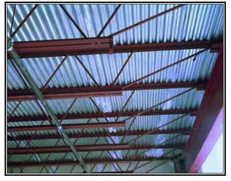
A concrete structural system was originally considered for the Hertel Avenue Apartments in Buffalo. However, a combination of concentrically braced and moment resisting steel frames proved to be both more economical and faster to erect. Shown at top is the traditional exterior of the building, while pictured above is a detail of the structure's steel joist floor system.
