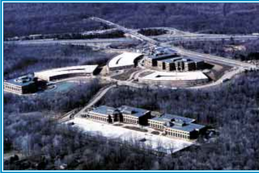
The four parking structures accommodate 3,600 cars and were designed to blend in with the rest of the office complex. Despite the large size of the project, the use of the Hybrid System enabled the parking structures to be designed and constructed in just 10 months.
