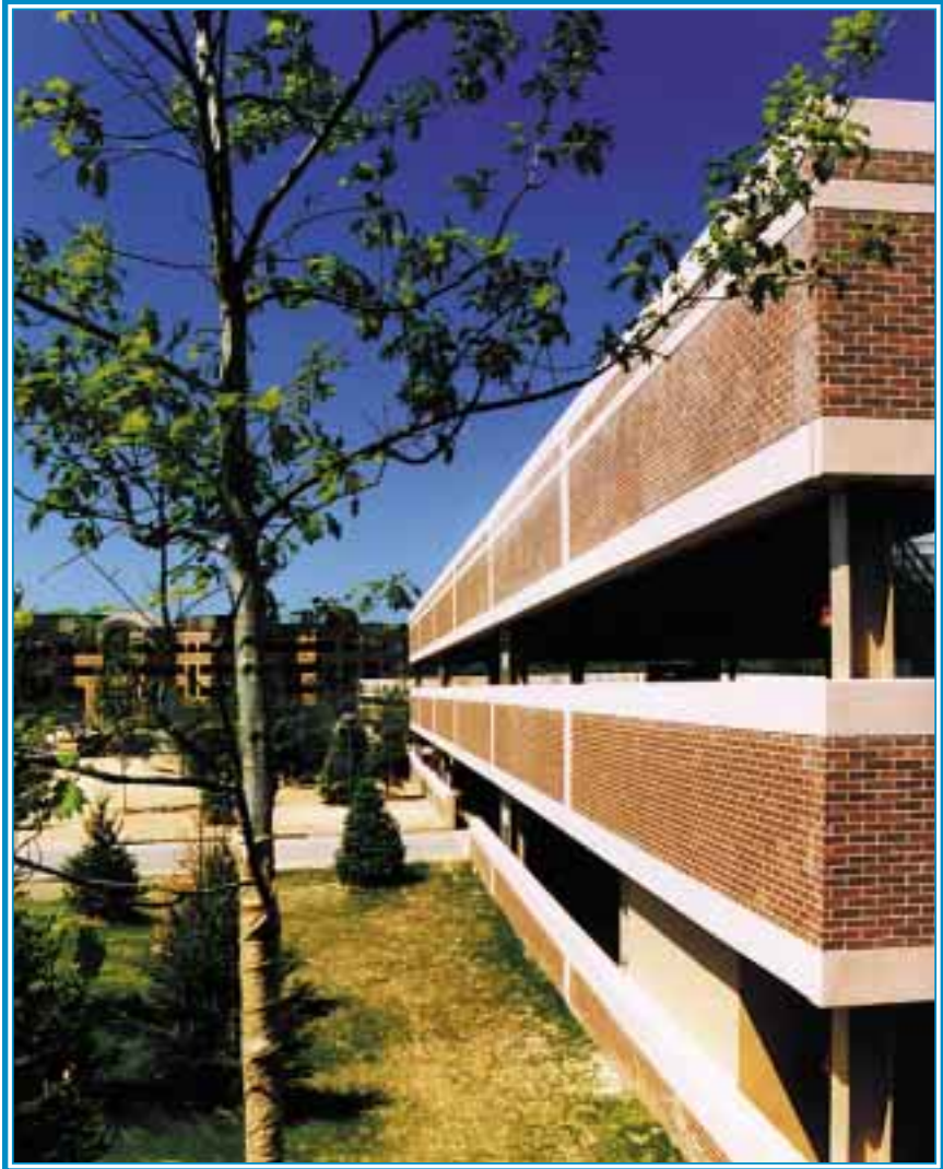
The guts of the Hybrid System for parking structures developed by Zaldastani Associates, Inc., are double steel columns supporting concrete tees. In this incarnation of the system, precast architectural panels incorporating a 2" brick tile were designed to be capable of supporting the precast floor units which spanned 60' from the interior column line. The spandrels, in turn, were supported on the steel columns.
