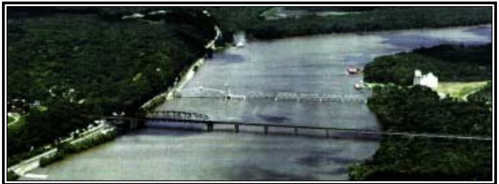
The new U.S. Route 36 Bridge is in the foreground, the old is in the background.
