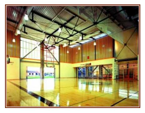
The architects left most of the steel frame exposed in the gymnasium both to express the building's structure and to create a more open design.
