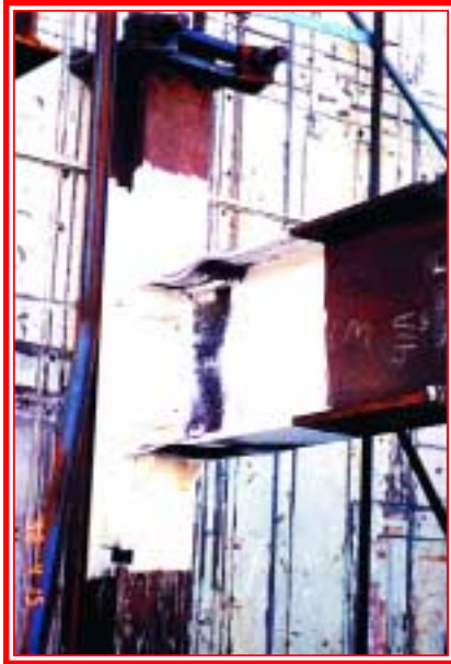
Figure 14: Hinging and buckling at +7 Delta yield for the W36x280 beam
