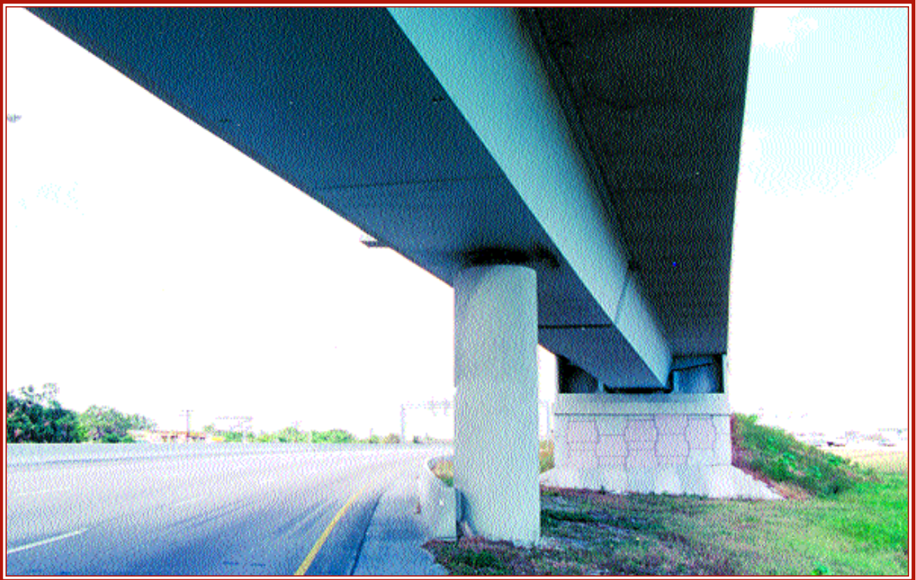
A steel box ramp near Miami
