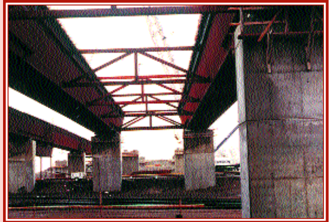
Macmillan Yard Bridge in Toronto
