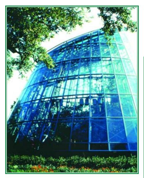
trusses arranged radially around the perimeter of the glass enclosure. All truss chord and web elements were designed using shopwelded pipe members to improve reflectivity of sunlight, minimize maintenance requirements, and eliminate the sharp edges so dangerous to butterflies. The slender perimeter trusses, which are spaced on 16' centers at the exhibit base, utilize 4"-diameter pipes for the vertical chords and 2"-diameter pipes for the web members.
