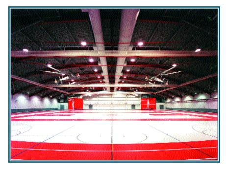
isfy the School Board's desire to minimize the volume and the new building and thereby reduce heating costs. The solution was a curved roof supported by exterior structural steel elements and clear-spanning 170' over the field
