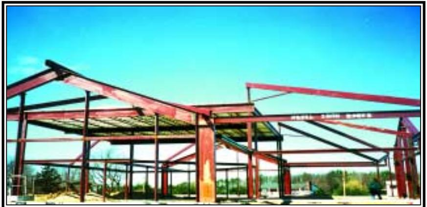
*Properly designed structural steel frames will not only reduce costs, but will also allow for future expansion.*
