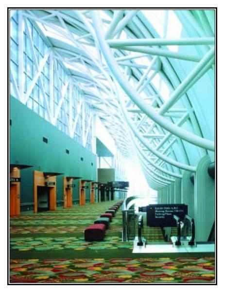
The main concourse features "banana" trusses on one side and "snowflake" X-bracing on the other.
