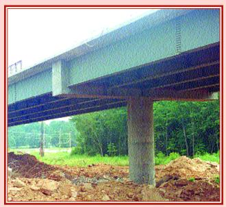
tensioning was applied utilizing transverse bars placed in the deck. The post tensioning was distributed over an effective slab width, considered to act with the cap, to insure compression—from the top of the slab to the bottom of the cap-under all loadings.
