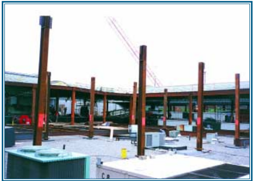
Shown are the column stubs and the new second level columns and framing in progress above the existing roof
