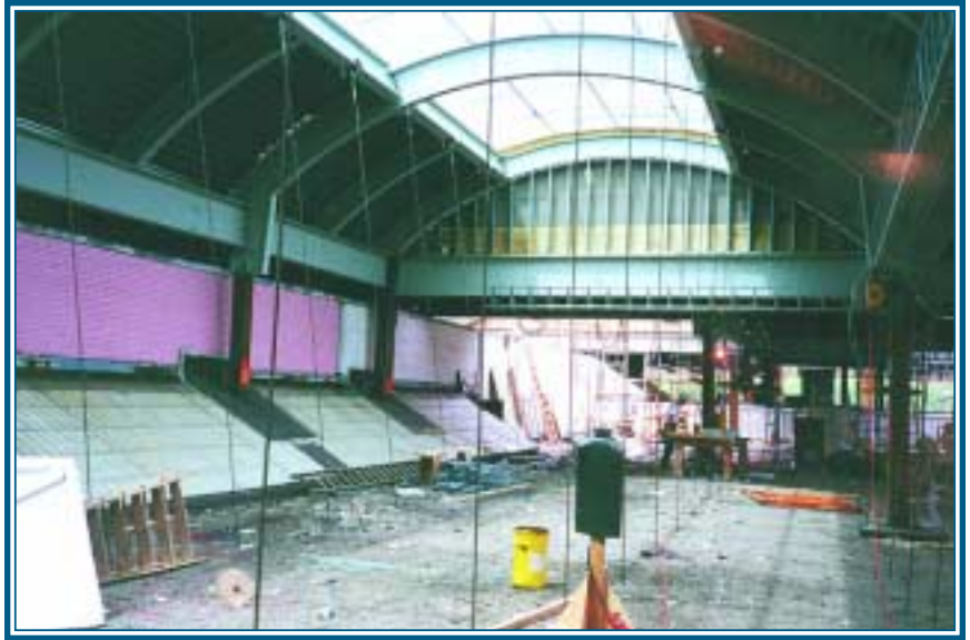
Shown is the second level framing and skylight above a workplatform installed over the existing mall first floor
