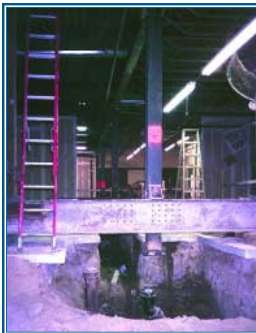
(Top) Typical basement area work scene for column/footing upgrades
