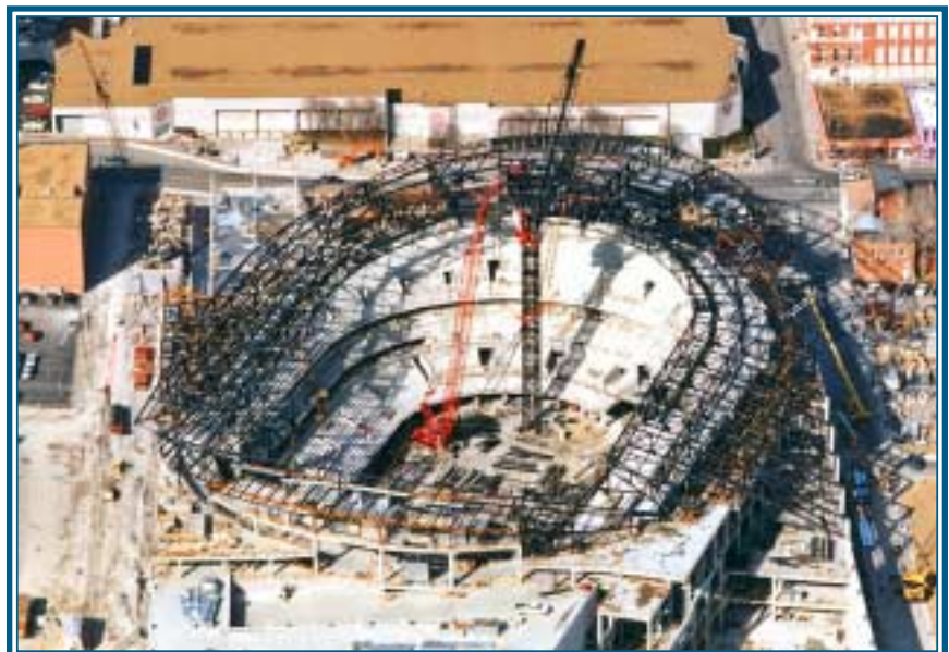
Photo by Phoenix Aerial Photography
