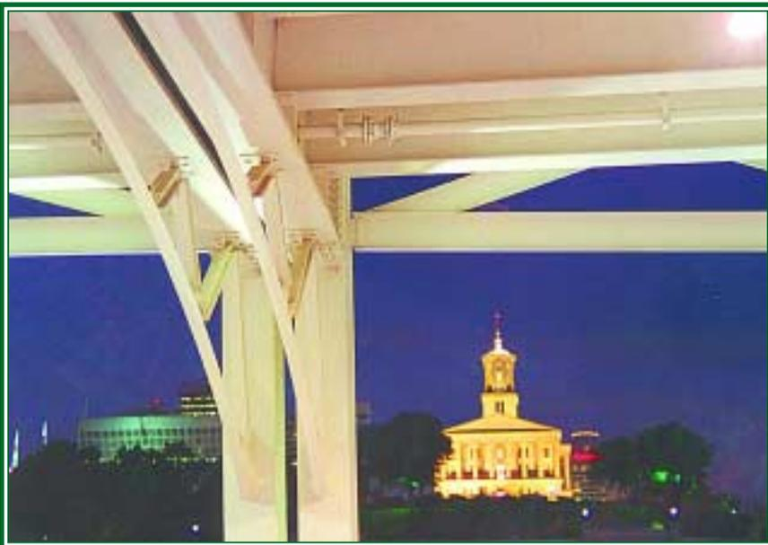
*A double bent at bay 7 provides an expansion joint that reduces maximum column tip deflection and secondary forces. William Strickland's 1850 Capitol Building glows in the background.*
