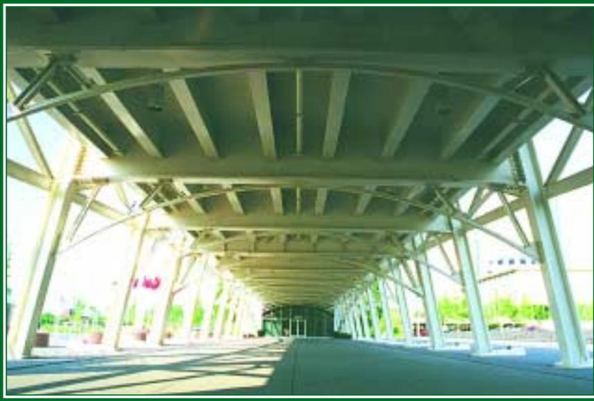
*The trestle is a series of simple spans carried by bolted moment frames. The decorative arches under the plate girders echo the form of the longitudinal arch.*
