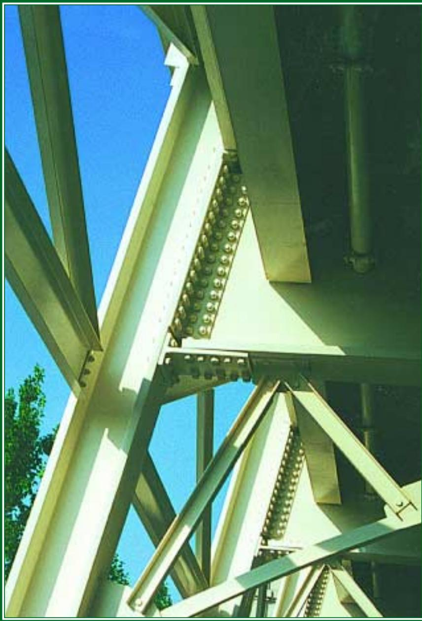
*Split tees and double angles connect the welded plate girders and rolled columns.*
