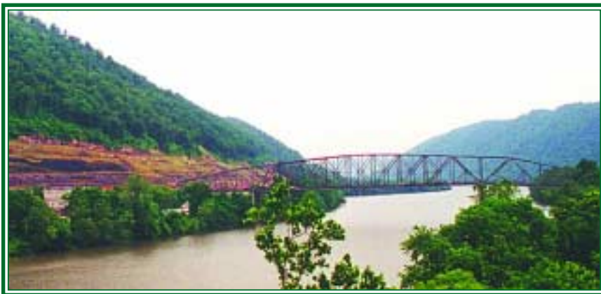
Pictured at top is the new bridge looking northeast. Note the T-intersection span in the foreground (painted white). Pictured above is the old Chelyan Bridge, which was built in 1929 and was posted at 29 tons.
