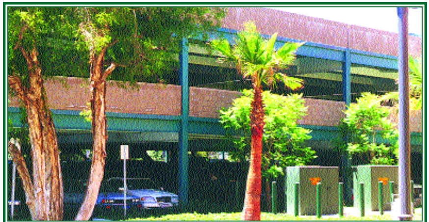
The parking structure design is simple, though attractive. It features concentric bracing for lateral stability, hollow structural section columns for aesthetic appeal and wide flange beams.
