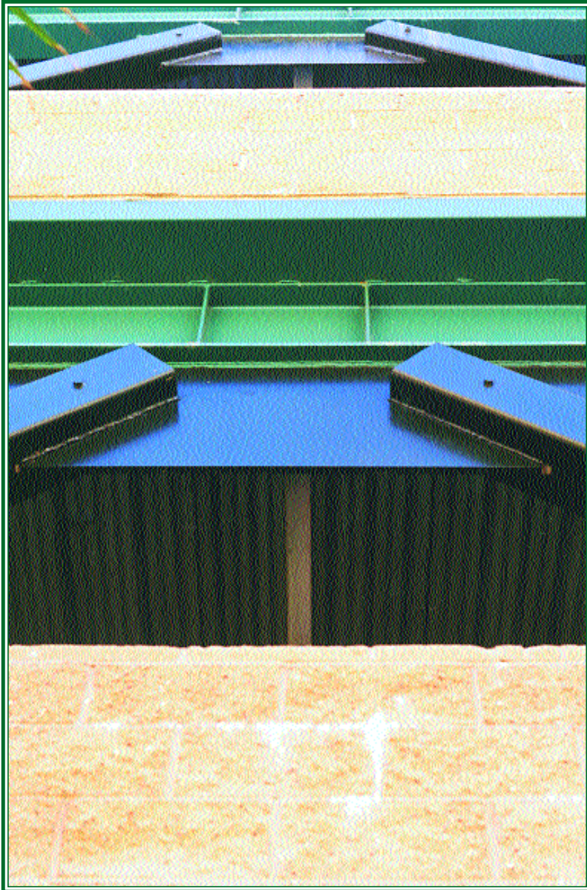
The parking structure design is simple, though attractive. It features concentric bracing for lateral stability, hollow structural section columns for aesthetic appeal and wide flange beams.
