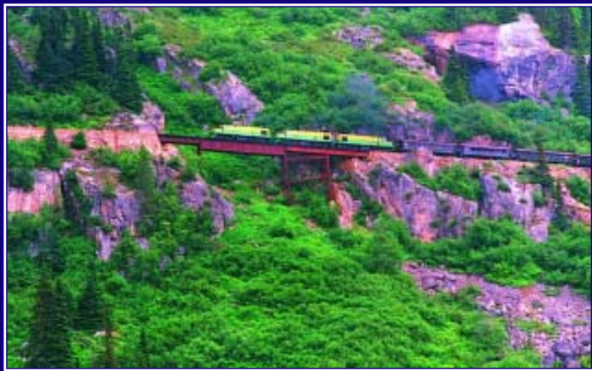
During a routine annual inspection, it was discovered that the seven-span, tiber trestle bridge 12A (top) had suffered mechanical damage. It was replaced with a new steel girder bridge (middle), which was installed in the fall—after tourist season was over. One of the major challenges faced the project team was the remote location and difficult site conditions. Bridge 15A (above) is located amid steeply sloping terrain. Though the steel bridge has been damaged by rockslides several times, it has always been quickly repaired—and some of its original, 50+-year-old riveted portions remain.
