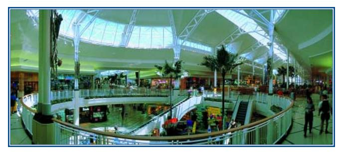
tuate either end of the retail spine add clarity and definition to the main retail precinct. Volumetrically, these courts are rendered as simple conical forms with the twin column supports being the only exposed structural elements. Daylight is introduced through a small oculus skylight at the pinnacle of the cone, providing both a dramatic and economical source of light.
