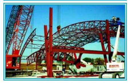
the space frame/skylight are resisted at the top of the radius counterfort retaining wall. This 18' high wall permitted construction of grades that establish the museum's entry at an observation deck level. This deck employed a conventional steel frame with composite steel metal deck and lightweight concrete fill. It extends into both hangars so that visitors can view the aircraft from an elevated perspective.
