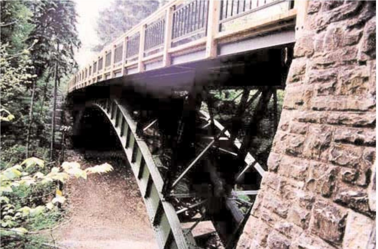
**T**he Bluff's Edge Bridge is a 140'-long steel arch bridge that spans a deep ravine along Lake Michigan in Lake Forest, IL. The primary structural system consists of three riveted steel arches supported by large stone abutments. Inclined (radial) steel columns support the deck structure above the three main arches. The original 20' wide deck structure consisted of 7 longitudinal (S10) stringers encased by an arched
