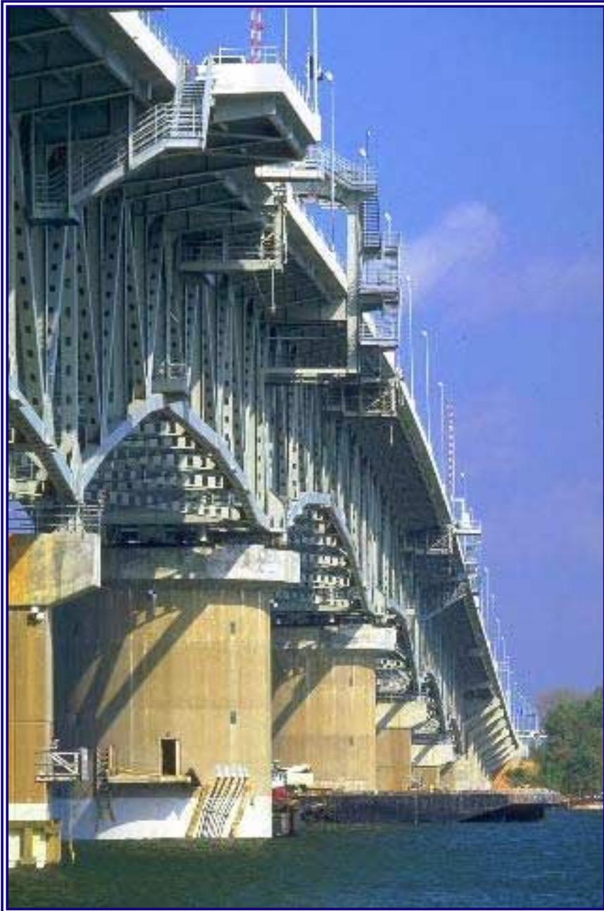
The Coleman Bridge in Yorktown, VA had to be redone if it was to meet the current and future needs of travelers in the area. The two-lane, 26'-wide bridge was replaced with a completely new 77' wide, four-lane structure – making it one of the largest double-swing span bridges in the world. The bridge, which has four 12' traffic lanes and two 10' breakdown lanes, is supported by the existing river caissons.
