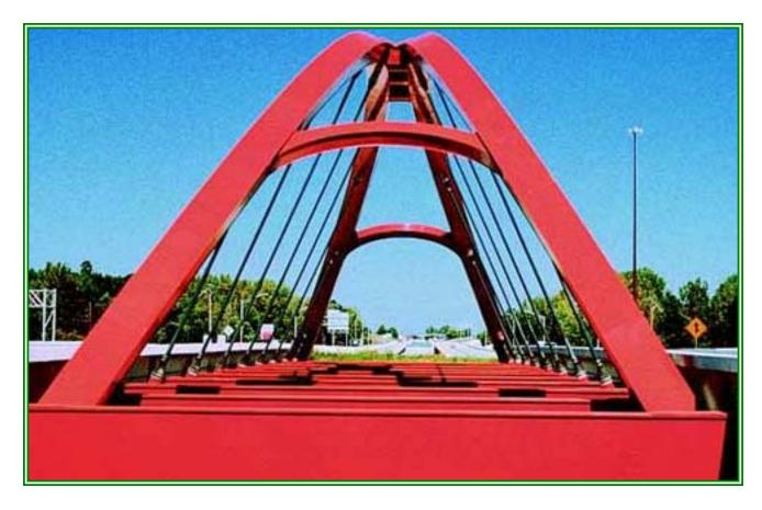
redundancy of the structure. The innovative composite deck system consists of a biaxially posttensioned, cast-in-place deck spanning longitudinally between transverse post-tensioned, steel box girders that are spaced at 19'-9" centers. Post-tensioned concrete structural parapets stiffen each edge of the decks. The 137'-long transverse girders are supported by cable-stays located in the plane of the arches and cantilever 48' outward from the stays.
