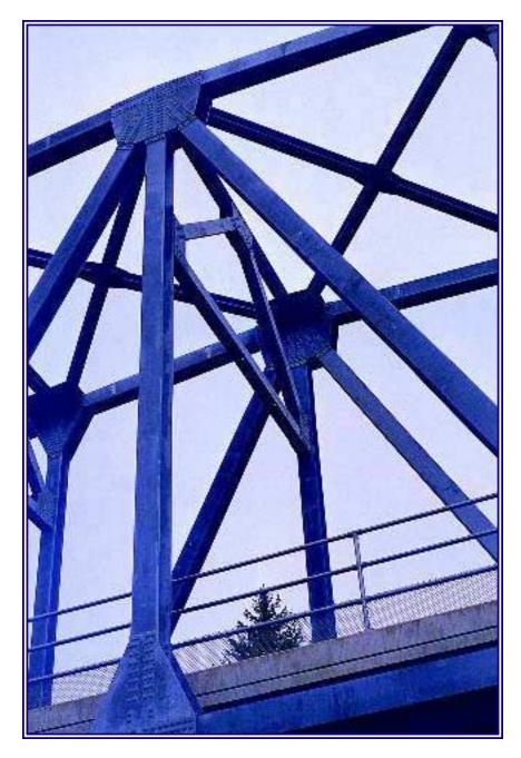
leading to a final structure design of a Modified Warren Truss. The following are some of the key design features: haunched top chord to reduce member sizes and improve the appearance; complete field assemble using high strength bolting; all truss members were designed using 14" rolled sections; the floorbeams were designed with a composite concrete ballasted deck to reduce live load impact and facilitate track maintenance.
