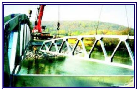
system, an analysis of the capacity of the elastically braced top compression cord, and full design and detailing of all connections. The design was in accordance with AASHTO Strength Design Methods, including provisions for slip critical connections.
