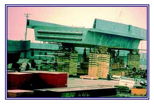
tions. The sections were staged on the east side of the freeway and crossed over during night erection. This could only take place in a tenhour window beginning at midnight on a Saturday night. A stiff financial fine was stipulated for each minute exceeding this time limit by the contractor. The first section was erected at the west abutment and allowed the team to practice for the erection over the freeway.
