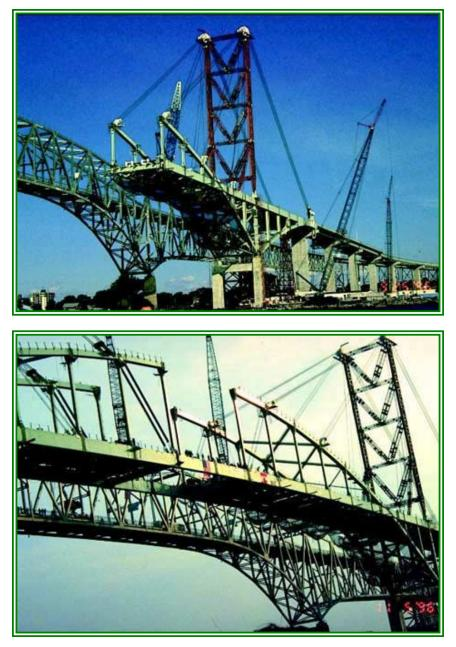
that provides the sole horizontal support for the entire arch. In addition, it provides most of the flexural resistance of the arch segments.
