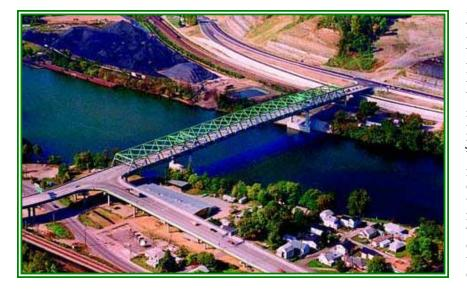
The new Admiral T. J. Lopez Bridge in Chelyan, WV is a modern four-lane bridge over the Kanawha River that replaced the existing deteriorated Chelyan Bridge. The new bridge is a three-span continuous, constant depth, through Warren truss with no verticals and spans of 247.5'-594'-247.5' (1,089' total). The poor span balance was dictated by physical constraints at either end of the truss.
