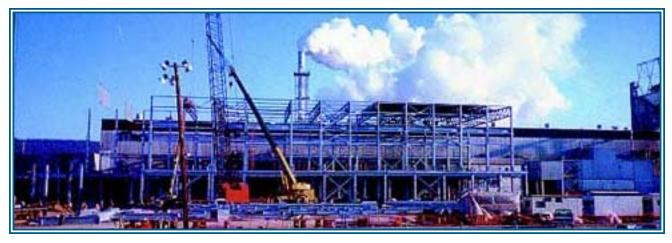
The S-2 Machine was positioned next to the S-1 Machine for efficiency reasons. For example, the same control operators could service both machines. Although the closeness of the buildings proved beneficial for the client, it posed several challenges for the engineer and constructor, such as avoiding large existing foundations and underground utilities as well as the actual physical tie-in to the existing structure. Furthermore, the S-1 Machine had not been designed with future expansion in mind.
