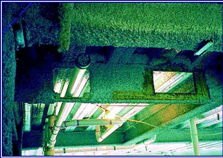
Web openings were utilized to accommodate many of the building's utilities.
