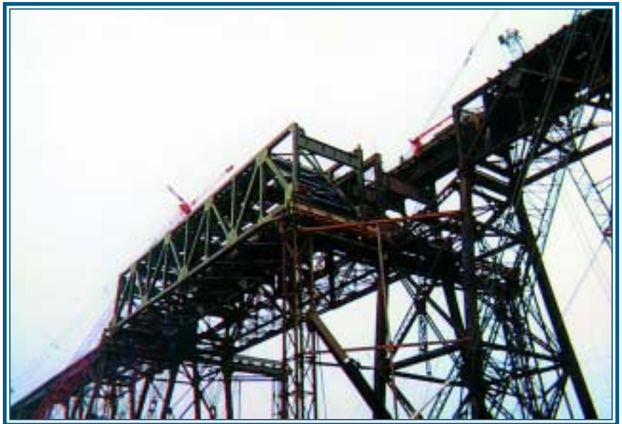
Pictured above and at top is the 180' truss during roll-in.
