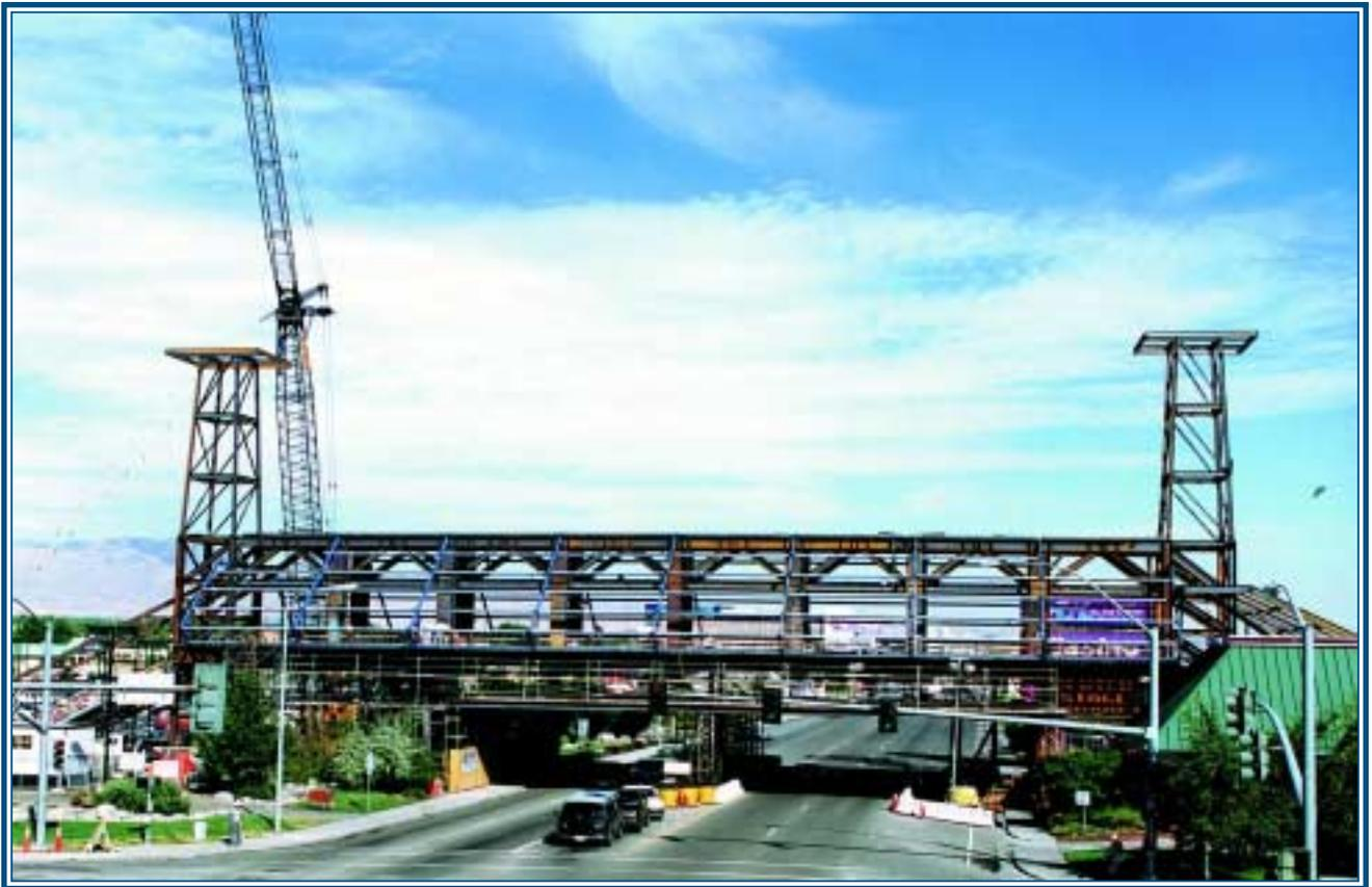
extra weight of a concrete structure would add to construction costs. In addition, the short window of time available for street closure demanded a structure that could be erected quickly.
