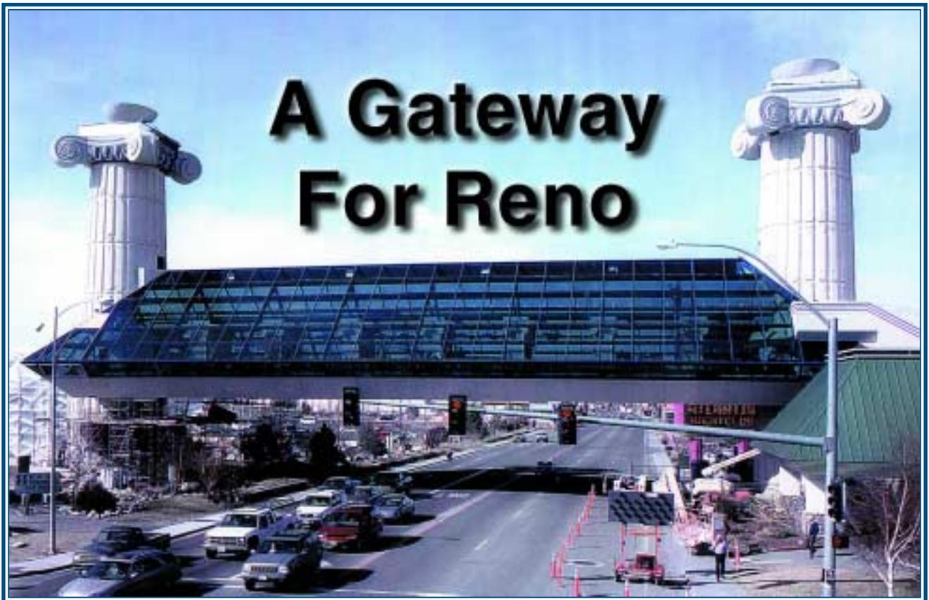
Composed of jumbo-sized steel wide flange members, yet retaining a light and open feel, the Skywalk at the Atlantis Casino and Resort combines a unique shape with structural ingenuity
