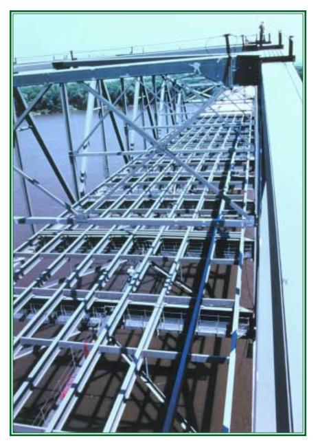
the truss span. The design live loading is HS25 with provision for 35 pounds per square foot future wearing surface. Based on the deck configuration, which may be altered to carry three lanes in each direction, a maximum of 2.34 fully loaded lanes of live load is attributable to each truss. Load Factor design was used in proportioning the members of the truss span, while allowable stress design was used for the slip critical connection design.
