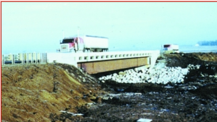
Pictured above is a creek crossing on Highway 79 south of Snyder, NE. The crossing is Nebraska's first use of the new HPS-70W material.
