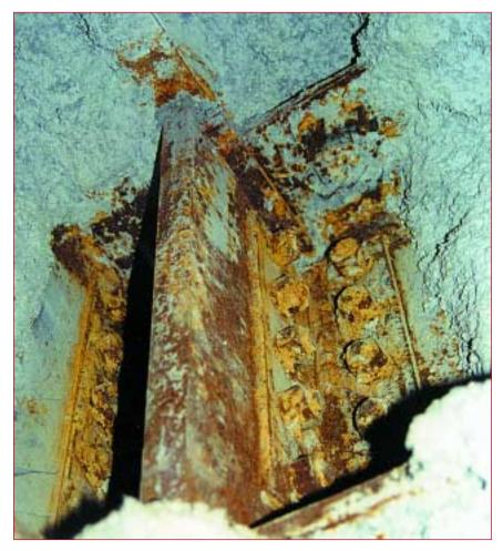
Figure 1: Typical exposure of fire protected moment connections.
