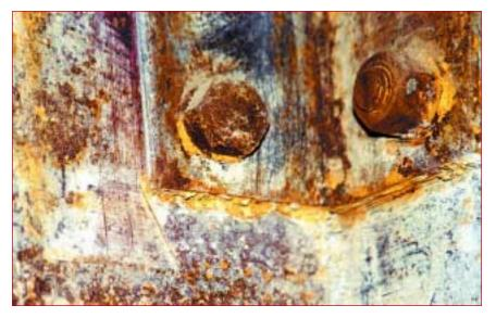
Figure 2: Complete removal of fire pretection at edge of bolted connection.
