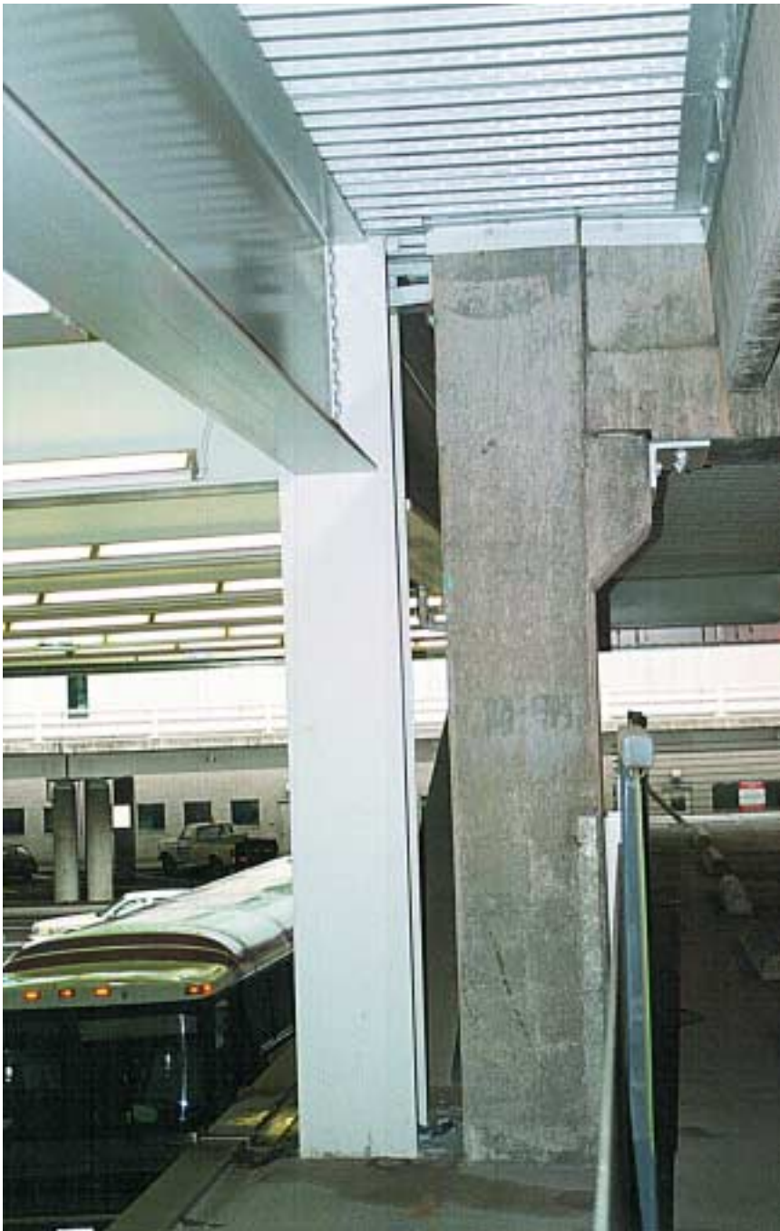
The addition to the existing parking structure at Portland International Airport included a 95' structure adjacent to the original construction as well as four new floors on top of the existing building.
