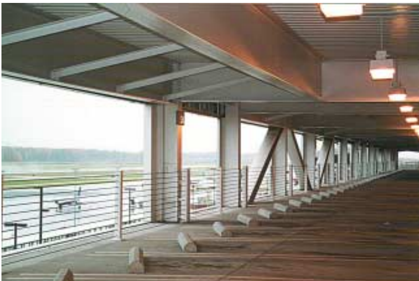
The new steel parking structure features large expanses of column-free space, which makes parking easier as well as providing a more open and airy feel for the garage.
