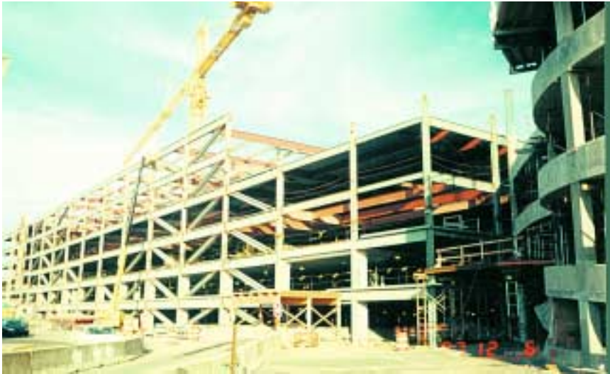
The expansion included added four levels of steel framing on top of the existing concrete structure.
