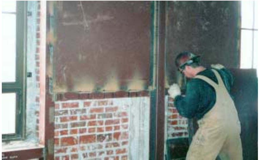
Shown above is the installation of one of the new steel plate shear walls, which were sized so two workers could lift one.
