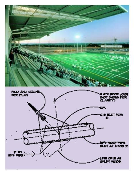
engineers designed a canopiedroof system that was completely independent of the stadium seating section. While the stadium seating area was being constructed, the roof was also being constructed in an adjacent field. Once the seating area was complete, the roof system was lifted into place and attached to 80 suspension rods and 16 uplift rods suspended from four steel towers.
