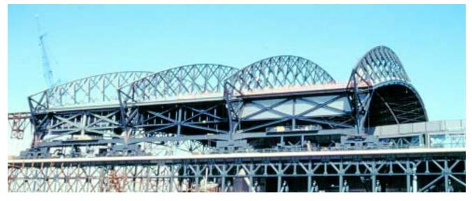
project schedule and design challenges. The retractable roof was designed for speedy erection and to minimize the impact on the construction of the seating bowl. The close proximity to the Seattle Fault required special seismic considerations, such as the use of an innovative viscous damping system in the roof that reduces the seismic forces by 50%.
