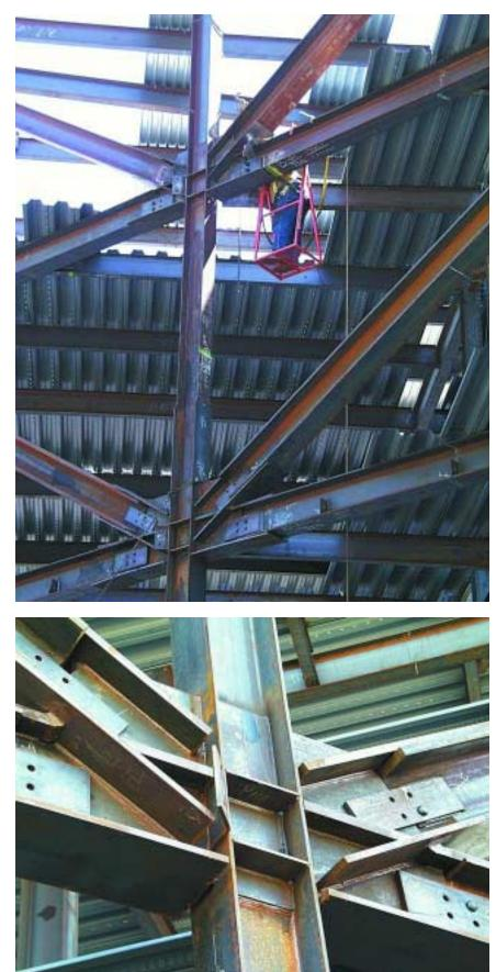
collaborated to create brace frame details that satisfied high load demands, simplified erection, and met budget and schedule requirements. Despite the high seismic load considerations, the final weight of the structural frame was less than 10 lbs. per square foot.
