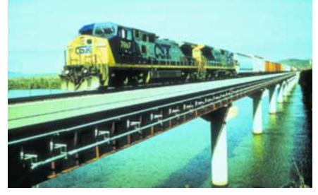
River is an economical and aesthetically pleasing design with low maintenance weathering steel girders and slender circular pier columns. It combines the required strength, function and serviceability with a clean slender appearance that blends well with the natural river environment and wooded riverbanks.
