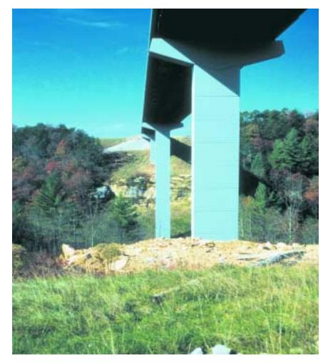
to erect. Stockpiled prices for HPS 70W steel for both bridges were \$0.30 per pound. The completed cost for the complete structure was \$95.34 psf.
