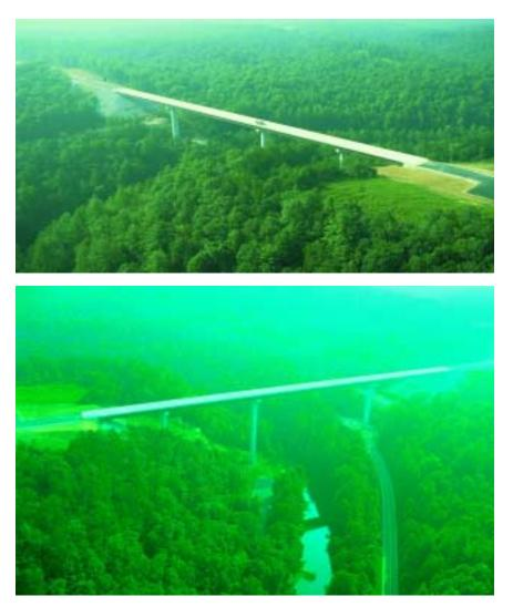
ituated in the Big South Fork National River and Recreation Area the bridge is a four-span welded plate girder structure with spans of 145'/220'/350'/280'. The superstructure is composed of four girders spaced 12' on centers, supporting a 42'wide composite concrete slab. Rising over 200' above the river, with only limited workspace for cranes, weights needed to be held to the minimum practical. Using HPS 70W steel helped achieve this.
