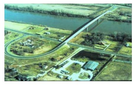
bridge was fracture critical. To provide redundancy, permanent cross-frames throughout the length of the bridge were designed to transfer the weight and live loading from one box to the other in the event that a girder section was cracked and became unserviceable.
