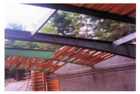
riveted frame was constructed with a haunched section. This not only provided a slender flowing profile, but it also mimicked the moment diagram of the bridge. This variable haunch allowed the design of the new frame to include a constant flange cross section over the entire length of the frame (including the vertical legs). This greatly reduced fabrication expenses by eliminating flange transition splices.
