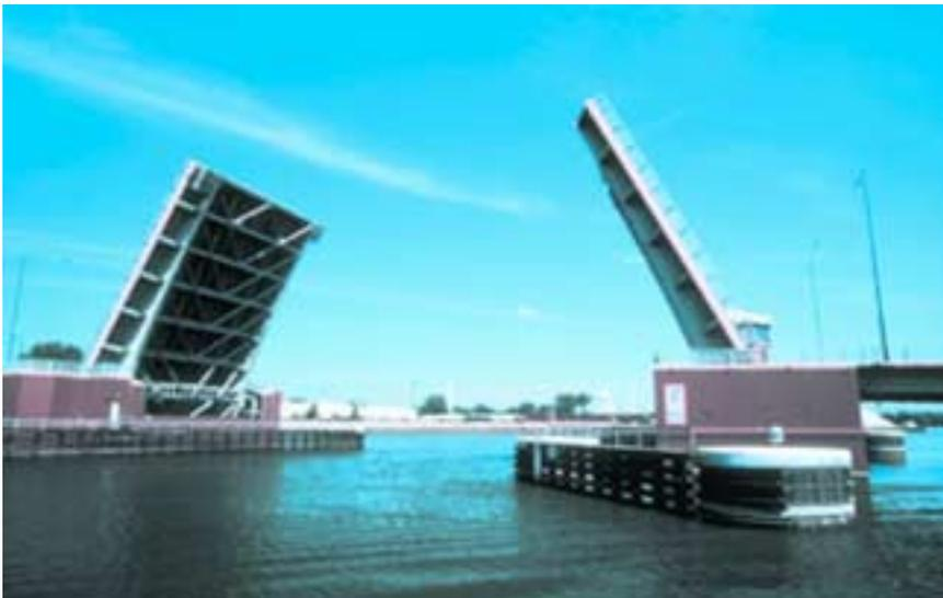
**T**he Main Street Bascule Bridge crossing the Fox River in Green Bay, Wisconsin, was experiencing ongoing, expensive machinery problems and increasing misalignment due to unknown foundation problems. Originally constructed in 1929 the bridge had become an historical landmark, however, in the summer of 1992, the City of Green Bay had
