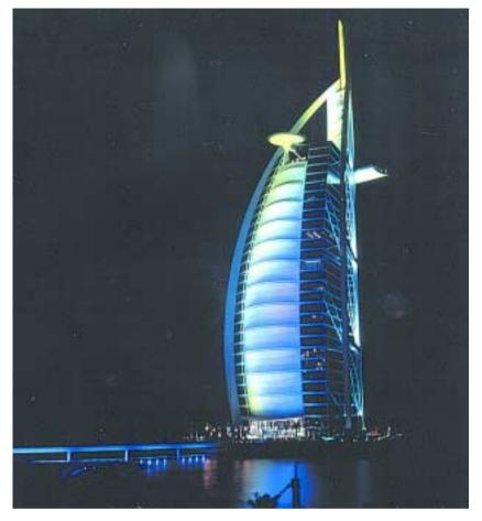
For the conceptual design, wind loading was based upon an extrapolation of the principles embodied in the UK Code of Practice for Wind Loading. However, in view of the size and unique shape of the tower, together with its proximity to the 100 m tall Jumeirah Beach Hotel, wind tunnel testing was undertaken for the detailed design phase.
