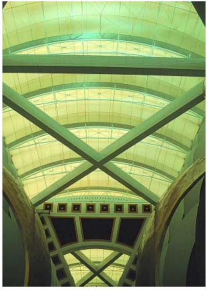
diagonal elements of the exoskeleton that, due to their design, had to be fully constructed before erection.
