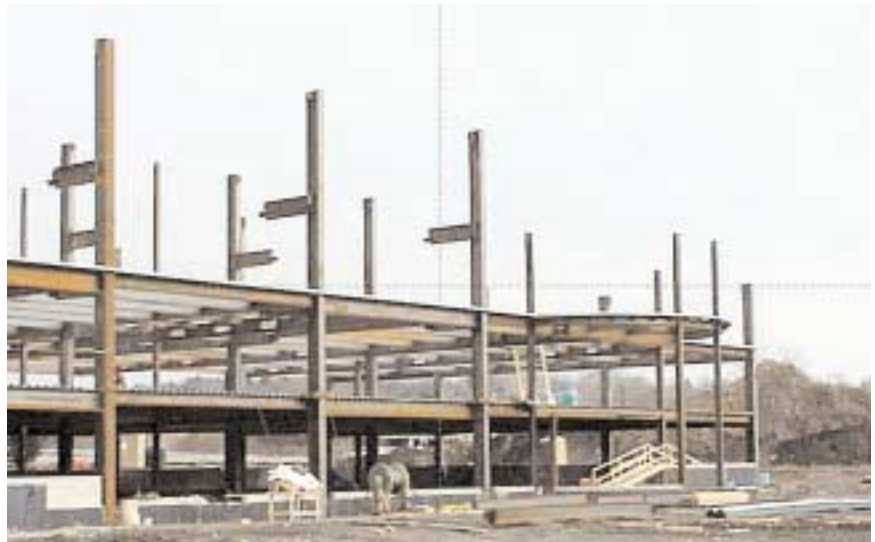
Wellesley Gateway Center under construction.
