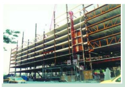
Advantages of Staggered Truss System include: • Improved layout flexibility due to elimination of interior columns & two-bay open space in longitudinal direction; • Large open spaces at base of building;
