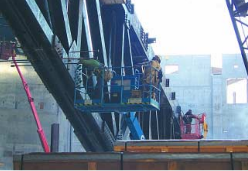
Field bolting match drilled connections.
