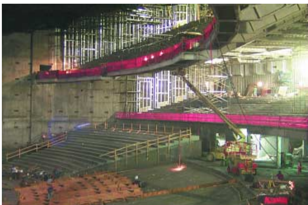
110 ft. cantilevered balcony.
