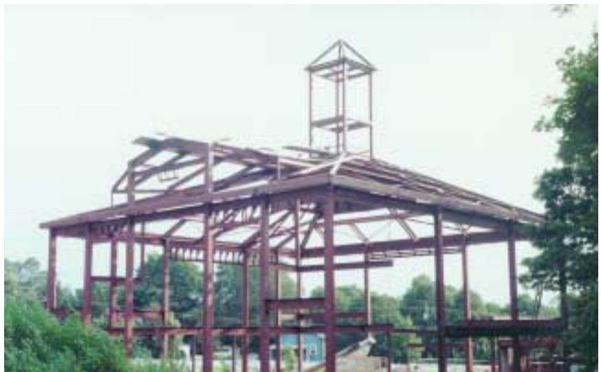
View of structural steel frame.
