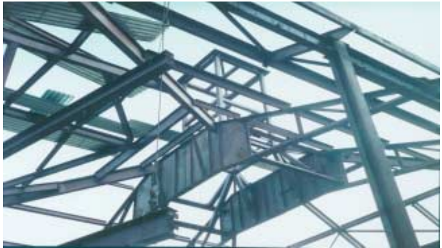
View of wish-bone shaped trusses at bell tower.
