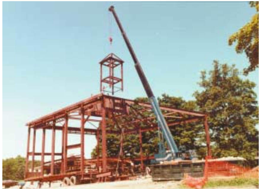
View of tower being erected.
